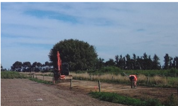
A drainage laser level was used to attain a 4% slope
