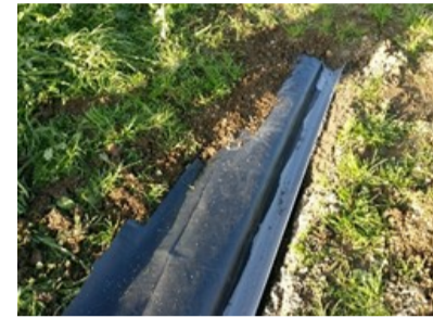
Cocksfoot, fescue and ryegrass mix was drilled into a levelled and sloped (4%) plot adjacent to the laneway. A 600mm deep drain was constructed to facilitate sampling of overland flow from the laneway
