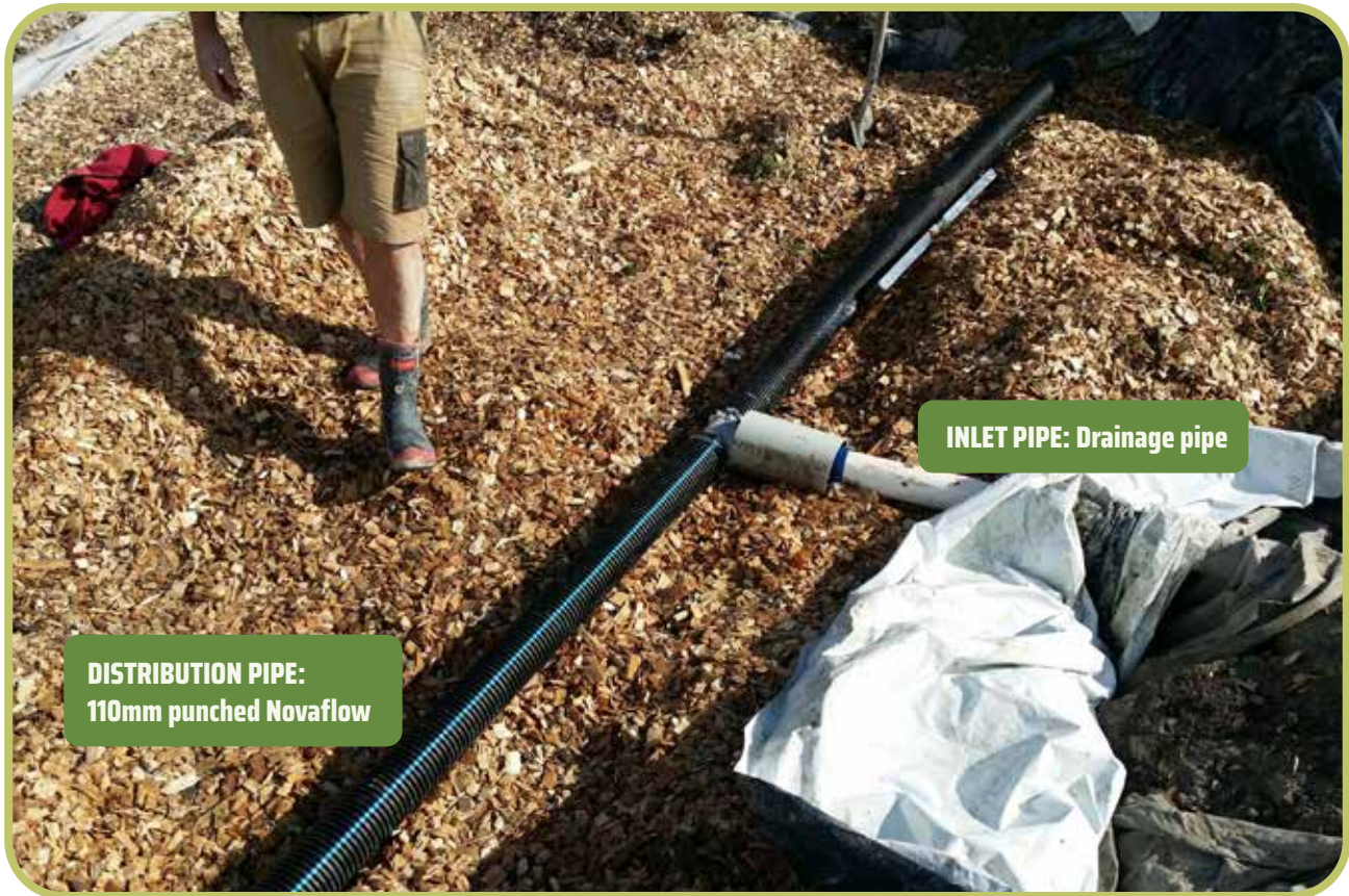
FIGURE 6 Arrangement of the Distribution Pipe at the inlet end of the bioreactor.
