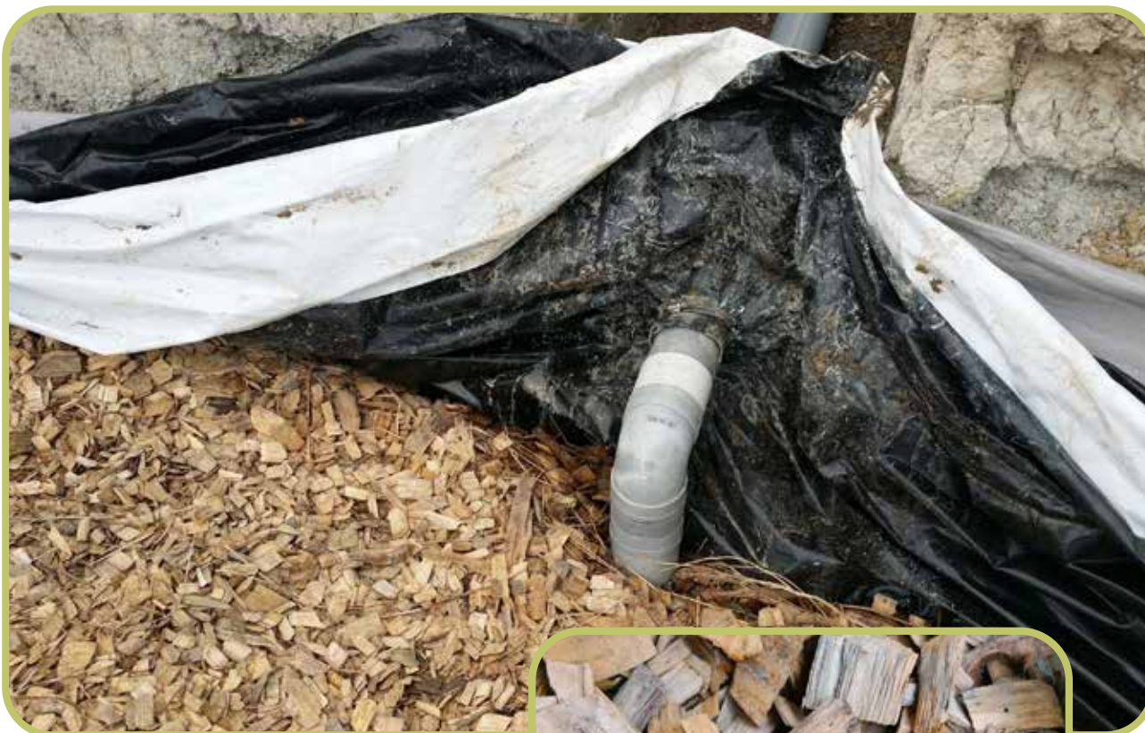
FIGURE 4 Shows the outlet pipe rising up from the base of the bioreactor and exiting to open drain.
