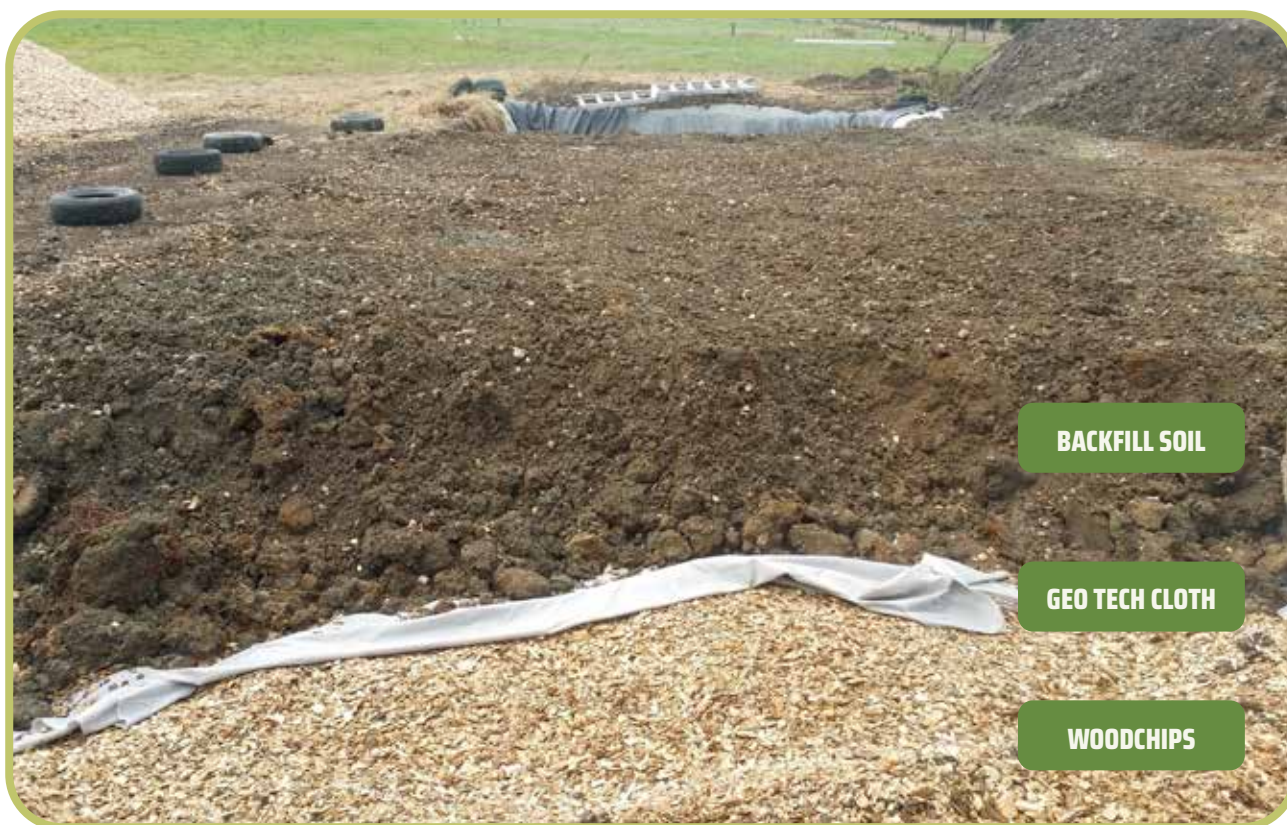
FIGURE 7 End view of bioreactor showing, Geotech cloth, woodchips and backfill.
