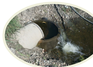
Inlet structure with overflow
