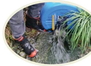
Wetland outlet, flow measurement weir with height scale
