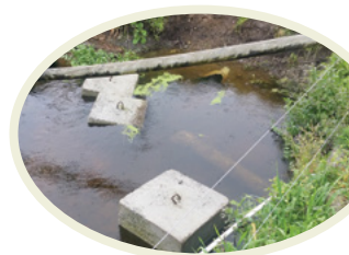
Submerged 160mm plastic inlet pipe with slots cut in
