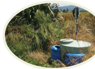
Wetland inlet, water height and orifice diameter control flow
